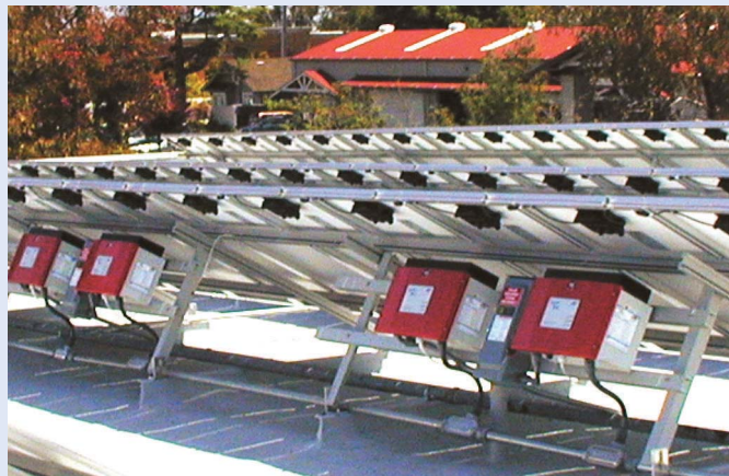
Rooftop Solar Array
