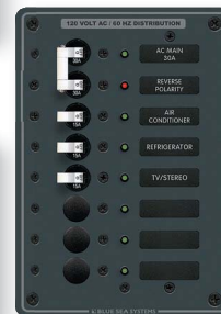
AC Main + 6-Position Breaker Panel
