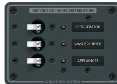
3-Position Circuit Breaker Panel
