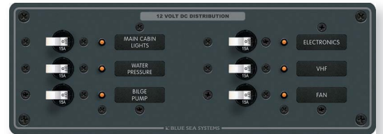
6-Position Breaker Panel
