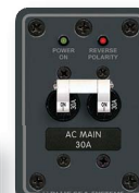
AC Main 30A Circuit Breaker Panel
